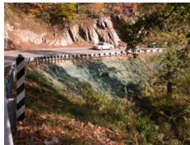
Above: A section of U.S. Route 58 in Patrick County which is recommended to be widened to four lanes.
